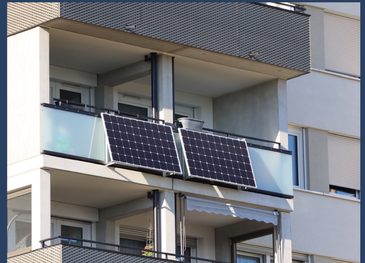
Two panels tilted on a balcony in Germany for better orientation. Photo: Sebastian Müller.
