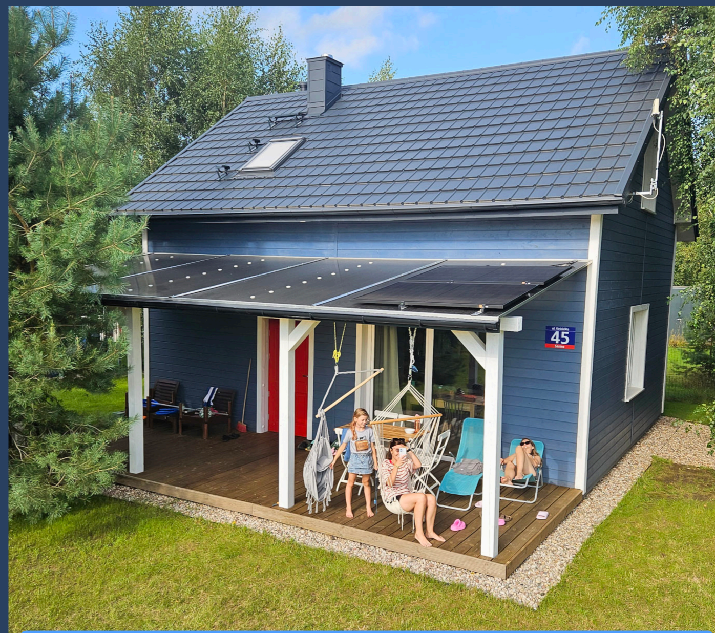
A PIPV system with two panels as a canopy over a porch at a cottage in Poland. Photo: OneStep.Solar.
