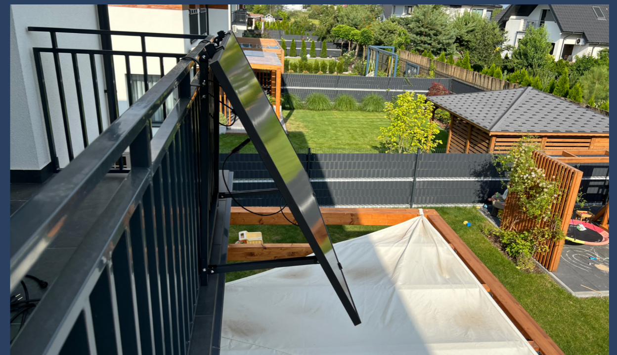
A panel tilted on a balcony in Poland showing the mounting system. Photo: OneStep.Solar.
