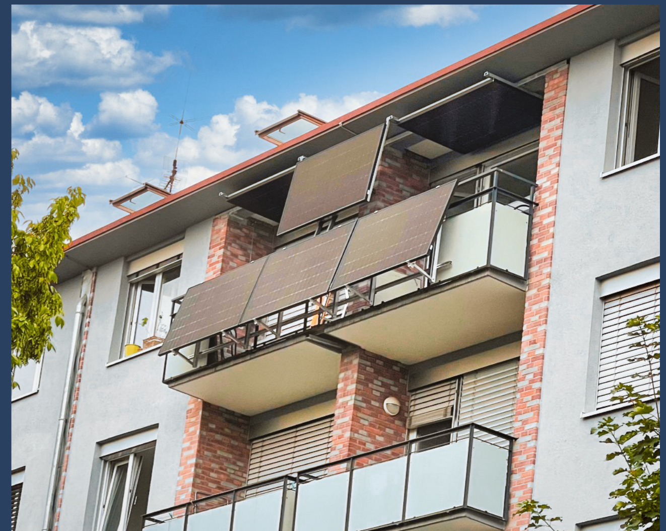
A balcony in Germany with three panels tilted on the railing and three retractable panels connected to the ceiling that can be used as an awning. Photo: Sebastian Müller.
